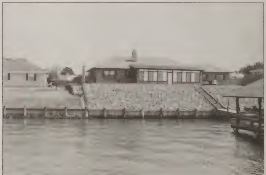
Bulkhead with revetment
